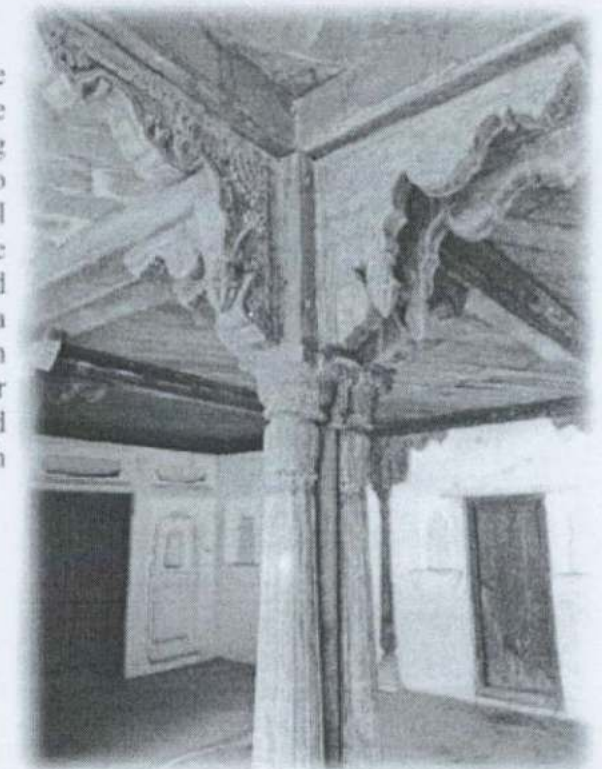
Interior view of Gohar Mahal
